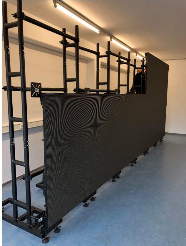
Ground Stack Installation
